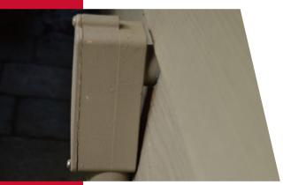
**HVAC systems -** these usually have some type of pipes and wiring that connect the outside unit to the inside of the structure and those points may not be sealed well. Any other similar locations like wiring boxes, vents, and utility lines should be checked and sealed.
